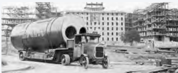
Queen Elizabeth Hospital under construction
