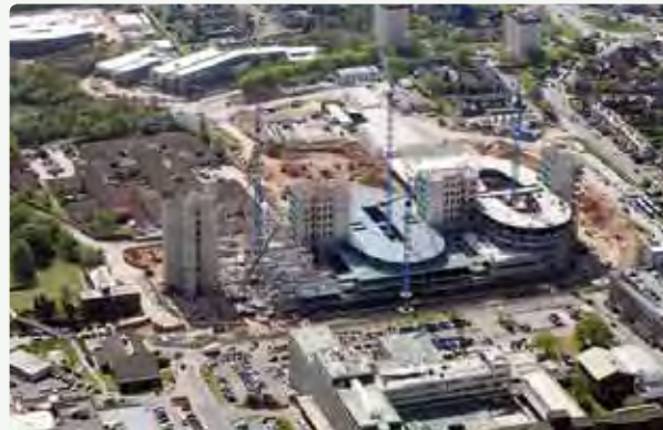
The towers begin to take shape
